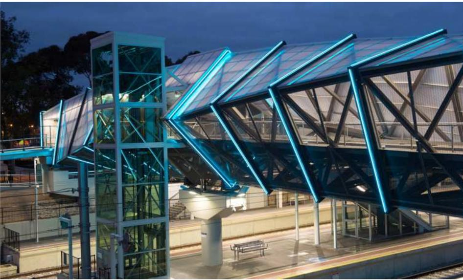
The overpass is a complex 50 metre long structure with a frame that twists 90 degrees over its length, built in collaboration with major engineering and construction firm McConnell Dowell.
